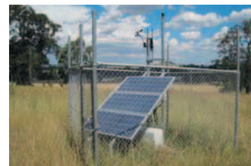
One of our seven real time noise monitors.
